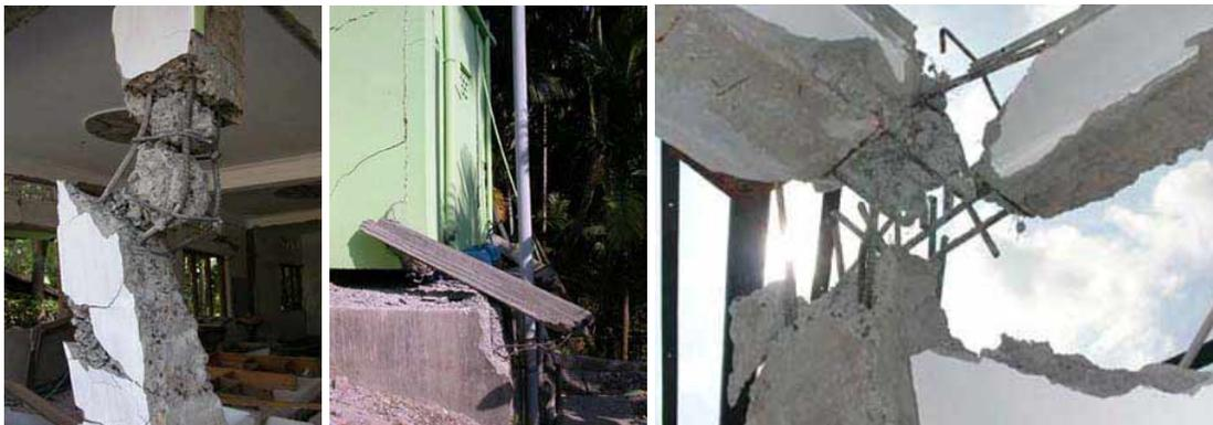
Figure 4. Poor shear design attributed to several column failures in buildings at Bamboo Flat.
