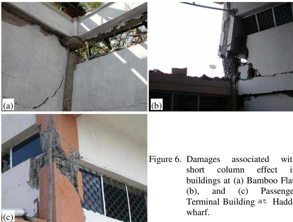
Figure 6. Damages associated with short column effect in buildings at (a) Bamboo Flat, (b), and (c) Passenger Terminal Building at Haddo wharf.
