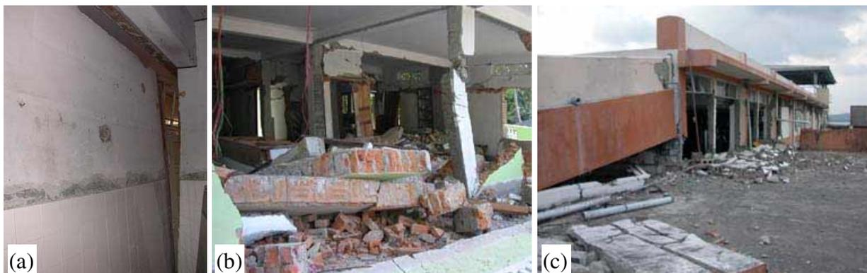
Figure 7. Out-of-plane failure of masonry infills in buildings at (a) Mohanpura (school building), (b), and (c).
