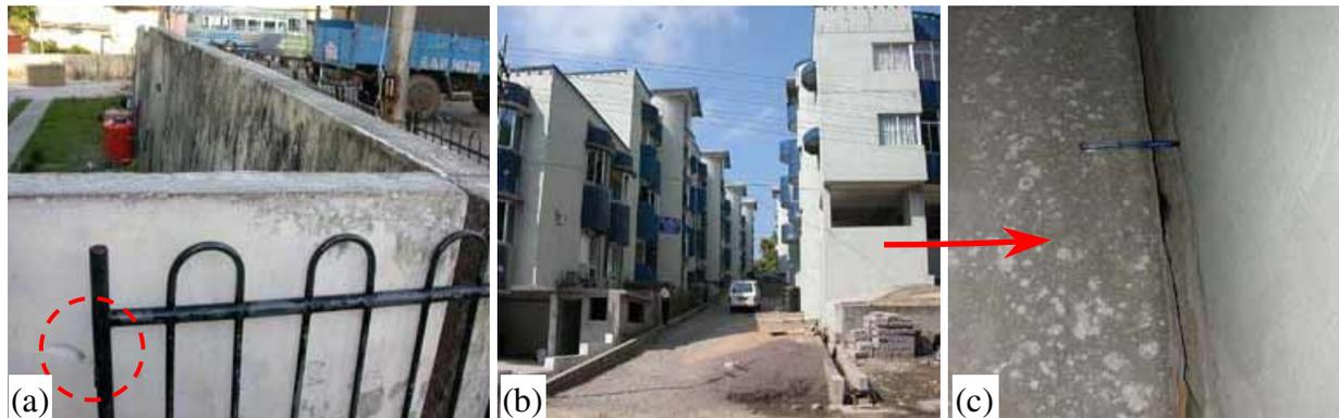
Figure 9. Ground sliding along slopes resulted in permanent lateral movement in (a) Police station building at Aberdeen Market, (b), and (c) residential building at Dilanipur.
