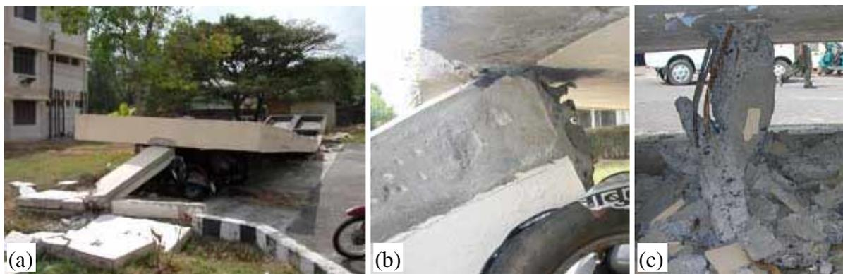
Figure 12. Collapsed RC scooter stand at Marine jetty office complex: (a) collapsed structure, (b) longitudinal rebars of at least two end columns were continued only up to soffit of the top beam, and (c) shear reinforcement was not present in at least one interior column.
