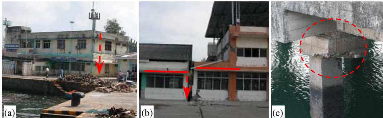
Figure 11. Foundation failure resulting into settlement of buildings (a) Operation Wing building at Marine Jetty, (b) Passenger Terminal Building at Haddo wharf, and (c) RC storage building at Haddo wharf.
