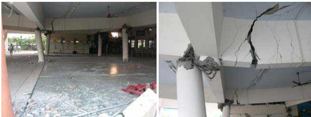
Figure 5. Severe cracking in RC members of Passenger Terminal Building at Haddo wharf.
