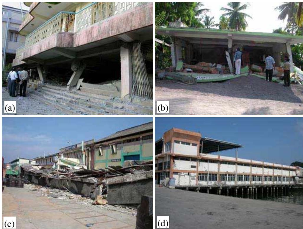
Figure 3. Collapse of RC buildings at (a) Naya Gaon, (b) Bamboo Flat, and (c) Haddo wharf, and (d) partially collapsed Passenger Terminal Building at Haddo wharf.
