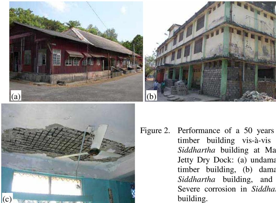
Figure 2. Performance of a 50 years old timber building vis-à-vis RC *Siddhartha* building at Marine Jetty Dry Dock: (a) undamaged timber building, (b) damaged *Siddhartha* building, and (c) Severe corrosion in *Siddhartha* building.
