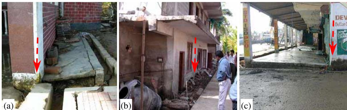
Figure 10. Settlement of several buildings at Bamboo Flat (a) 2-storey RC building, (b) 3-storey RC building, and (c) shopping complex.
