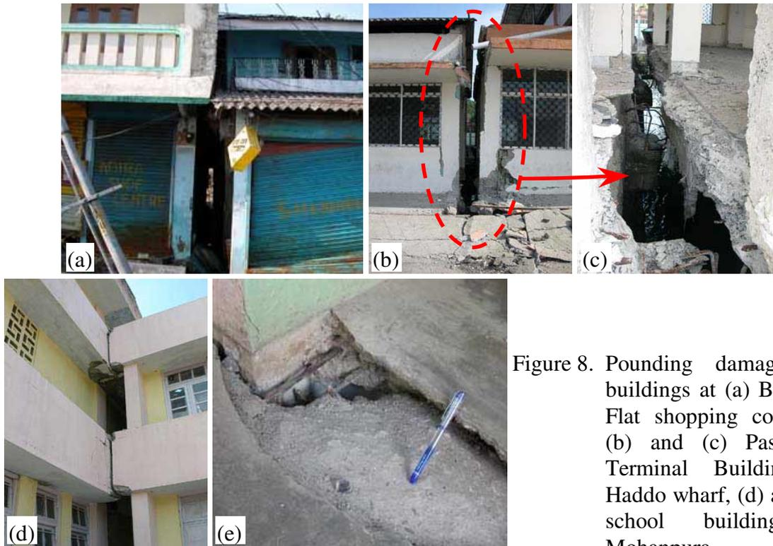
Figure 8. Pounding damages in buildings at (a) Bamboo Flat shopping complex, (b) and (c) Passenger Terminal Building at Haddo wharf, (d) and (e) school building at Mohanpura.
